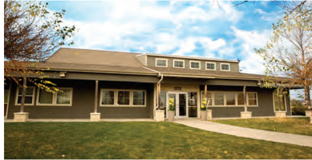
NORTH LOCATION – 3272 SALT CREEK CIRCLE
